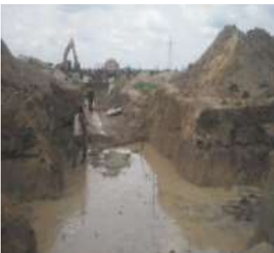
Plate VIII: Excavating timbering of trench wall.
