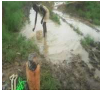
Plate XI: Fetching of dirty water for concrete mix.
